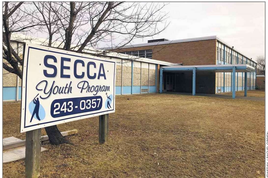
The George Washington School, more than four years after the town voted to sell it, nears demolition.
